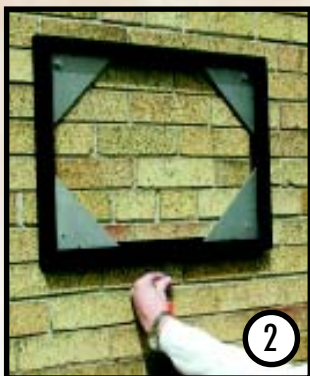
Remove security screw to release frame
